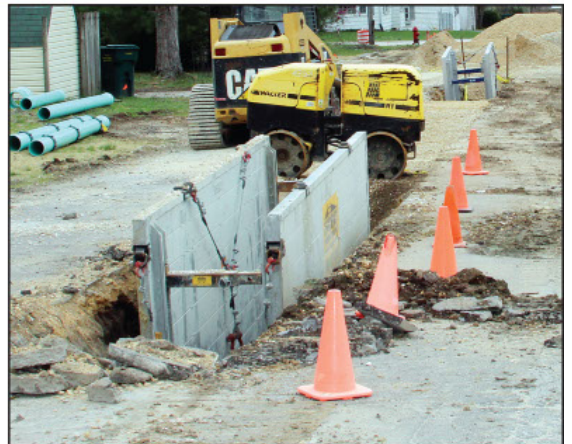
Above: work has started on sanitary sewer and water distribution lines that must be done before other work on the Georgia Street project. Right: Mayor Bart Niedner addresses people at the groundbreaking.
