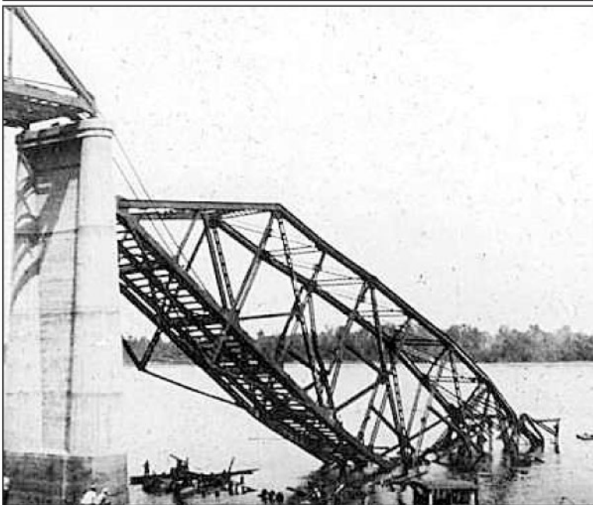
A span under construction on the Champ Clark Bridge collapsed on Sept. 6, 1927, killing one worker and injuring another. Despite the accident, work resumed two days later. (Photo courtesy of Betty Allen)
