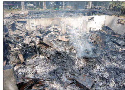
Fire completely destroyed the home of Joey and Christy Orf outside of Bowling Green last Wednesday night. Crews battled the blaze at the two-story home on West Outer Road for several hours. The Orfs and their children were not home at the time of the fire and discovered the flames as they arrived home just after 10 p.m. The family noted the outpouring of kindness from the community has been overwhelming and appreciated as they work to rebuild.
