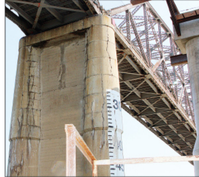
Wear is visible on the old piers that support the current Champ Clark Bridge that was built almost 90 years ago. Experts say the new bridge should last 100 years and will be more than double the width of the current bridge. Find more photos of construction online at www.thepoplestribune.com . Trib photo by April M. Frorick
