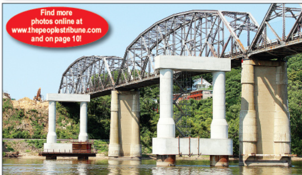
Media and local officials were invited to examine progress on the new Champ Clark Bridge on Friday, Aug. 3. Above, the concrete and steel piers are nearing completion across the span of the Mississippi River into Missouri. Steel girders are being set on the Illinois side of the river. In the background above, work can be seen on the retaining wall next to the Ayrco Convenience Store in Louisiana. Left: T. J. Calabatto, project manager for Massman Construction, discusses details of the $60 million project with individuals on a barge as it passes under construction and the present Champ Clark Bridge. By completion, the new bridge will be more than double the width of the present bridge that was built 90 years ago.
