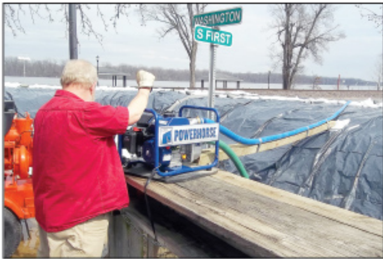
Mike Greenwell pumps seep water March 24 from the dry side of an earthen dam that's been built along part of First Street in downtown Clarksville. The dam is covered with tarp and sandbags.
