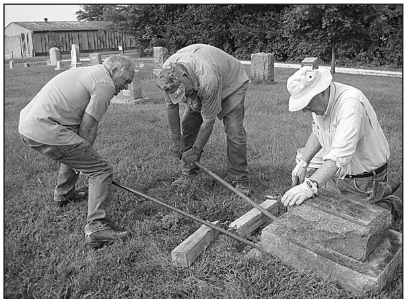
Workers level the smaller markers by using pry bars and filling in the low spots with gravel. The cemetery keeps a pile of gravel plus dirt to level sunken areas. Pictured are John Welch, Robert O Shea, and Dale Miller.
