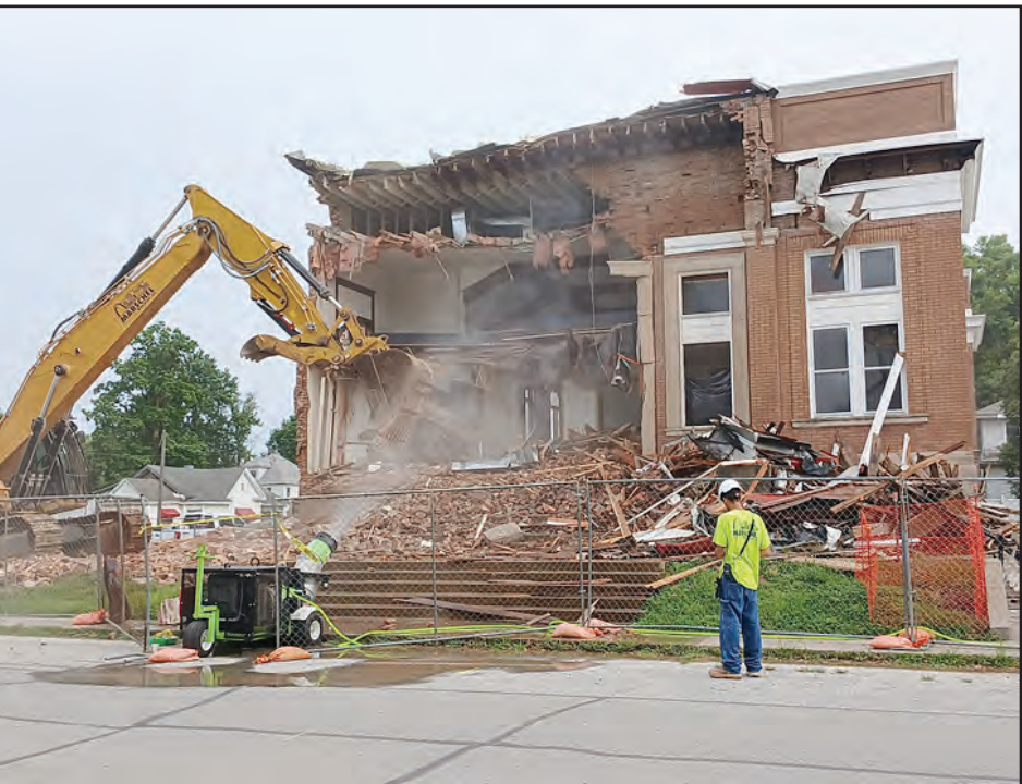
Second Baptist Church Demolition Pictured is the Second Baptist Church in Bowling Green during the demolition of the building. Plans are to rebuild a new church on the same location.
