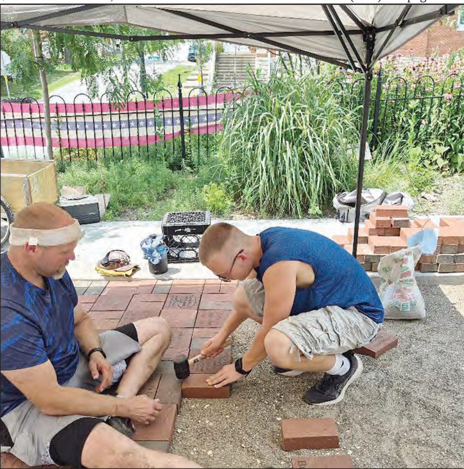
Pictured are pavers being installed at the Bel-Rose Park in Clarksville.
